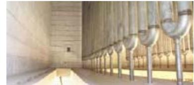
The two radiant modules are shipped with dimensions of 8m wide, 11m long, and 22m high, each weighing around 280 tonnes.
