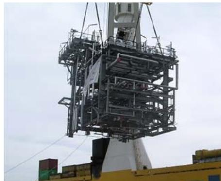
To meet the fixed heavy lift ship arrival time, the module yard had to meet a very aggressive five month schedule. Over 450,000 man-hours were expended to produce the pre-assemblies, complete with the instruments, wiring and all the testing and functional handover information.
