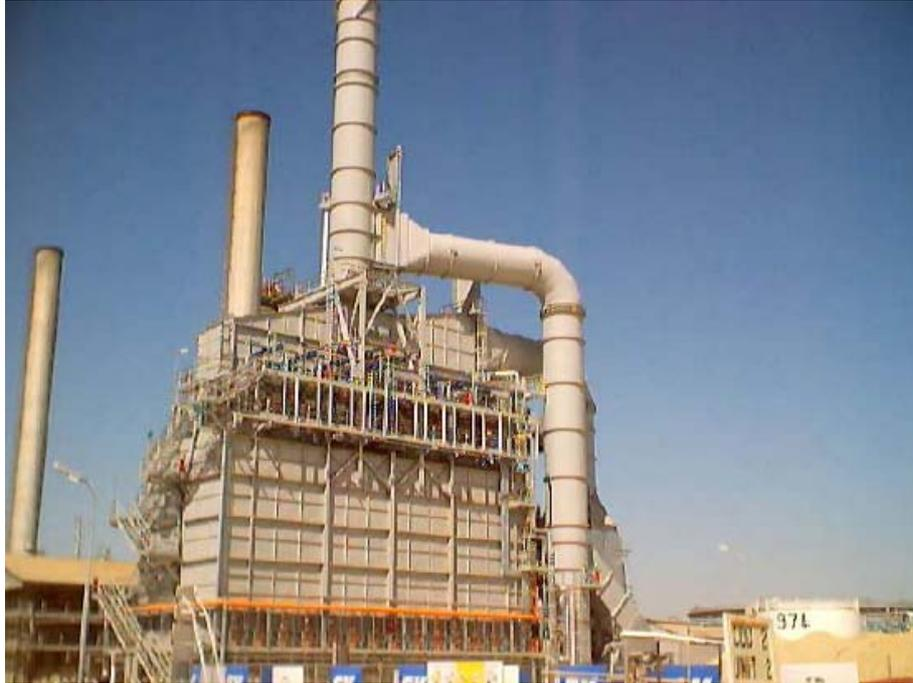
As part of Kuwait National Petroleum Company's (KNPC) on-going development plans for its Mina Al Ahmadi refinery, ABB Lummus Heat Transfer (LHT) was called on to design and install a new crude heater, to replace the existing Crude Distillation unit known as CDU#3
