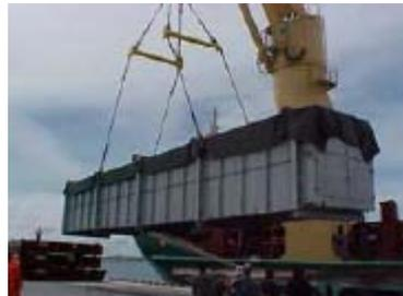
The larger of the two concrete lined convection modules was 25 meters long x 5 meters high x 5 meters wide and weighing 125 tonnes.
