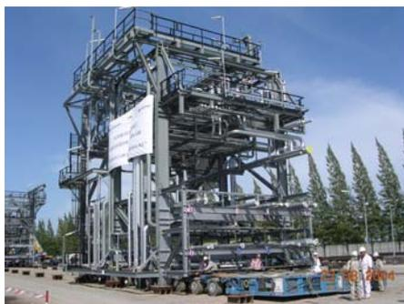
There were seven PAR sections, each weighing 150 tonnes, and two 250-tonne PAUs. Each PAR section was approximately 18 metres long by 12 metres wide
